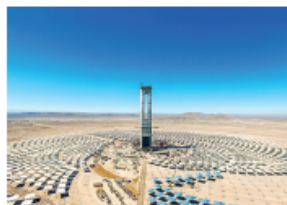
Solar Tower Receivers & Steam Generators
