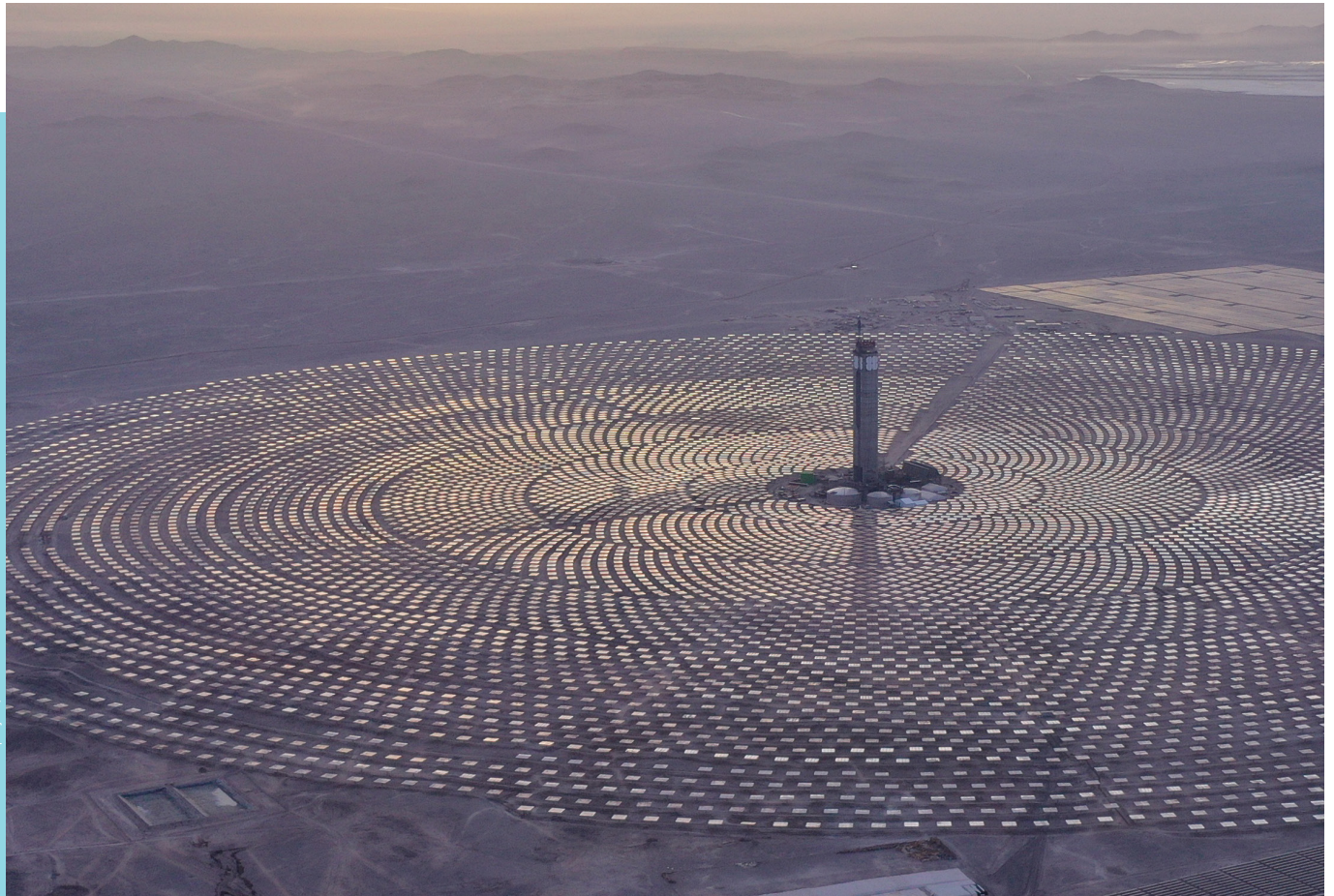
Credit: Cerro Dominador project, Chile
