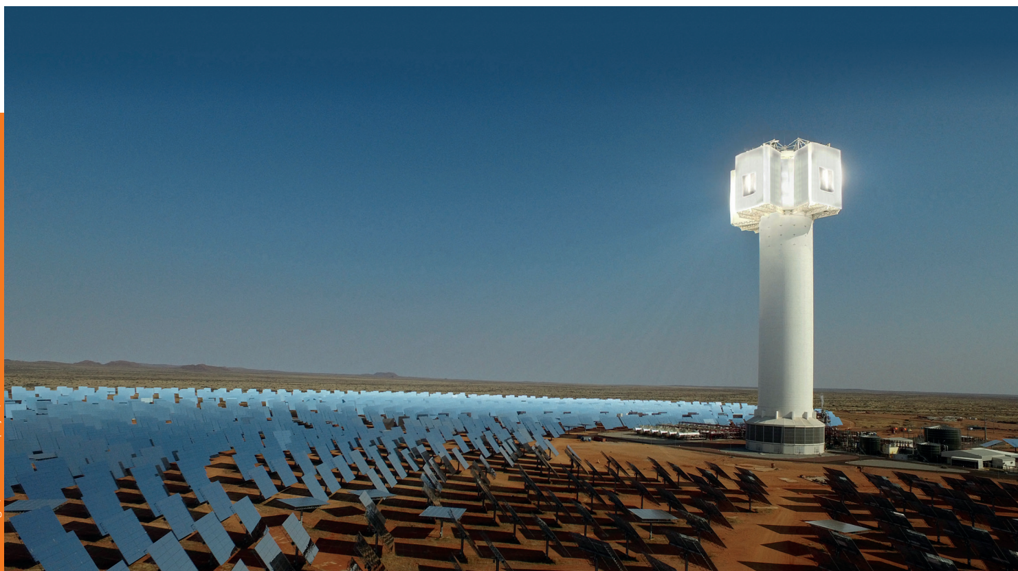
Credit: Abengoa, Khi Solar One project, South Africa
